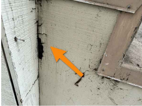
North West Stairs
